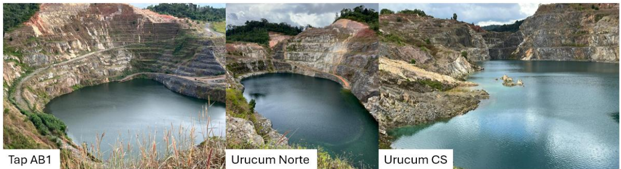
Figure 71: images of the open pits with water at the bottom observed during the visit. The image shows good geotechnical stability of the pit slopes.
