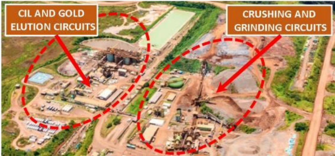
Figure 75: View of Crushing, Grinding and Processing Plants Source: Amapá Minerals, 2026
