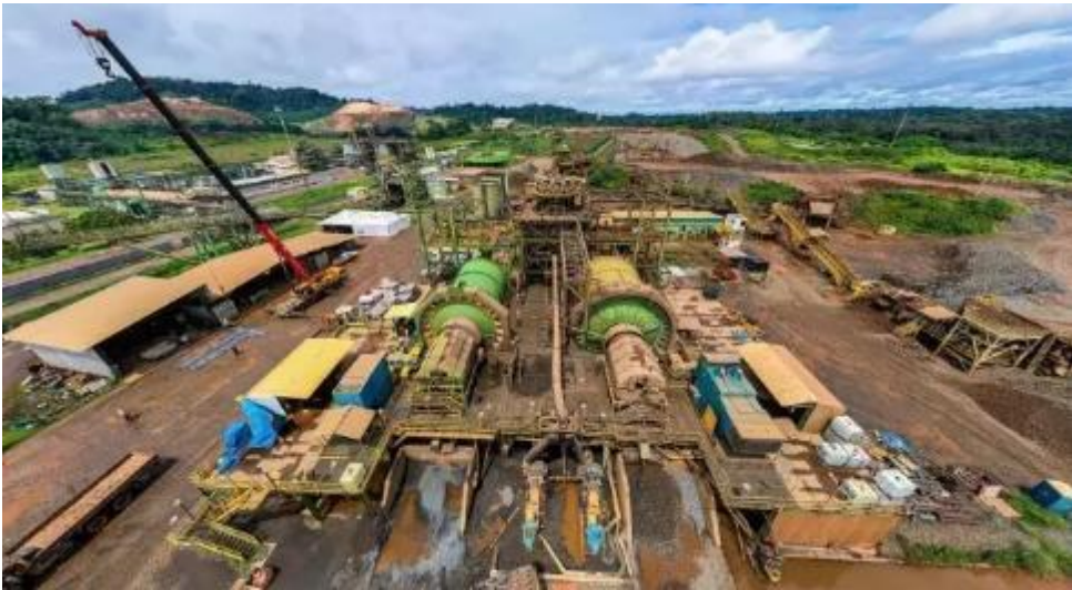
Figure 76: View of Grinding Circuit Source: Brasil Mineral
