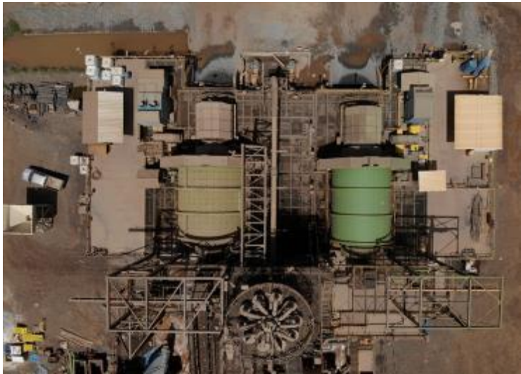
Figure 73: Top View (Processing Plant) Source: Cleber Barbosa
